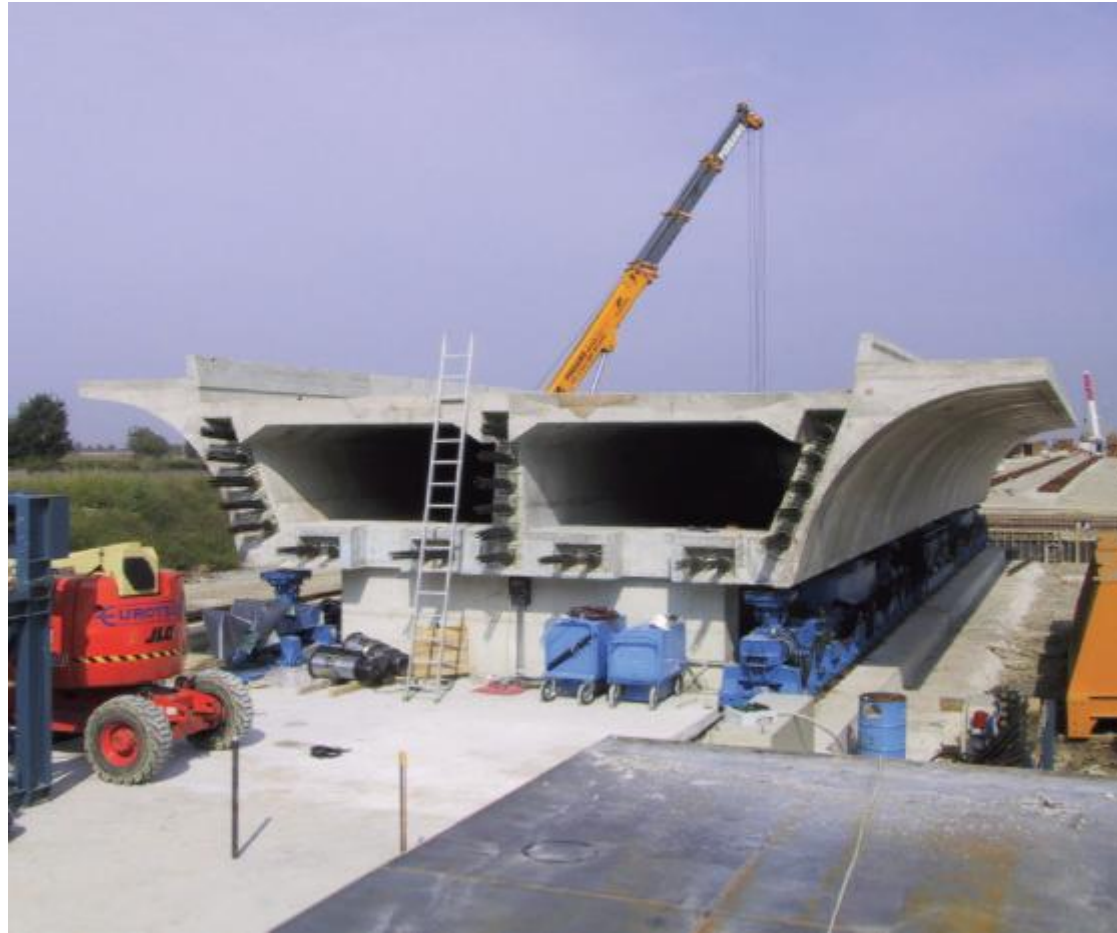
TWIN CELL BOX GIRDER
