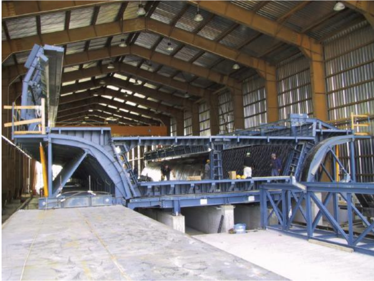
THE PRECAST AREA
