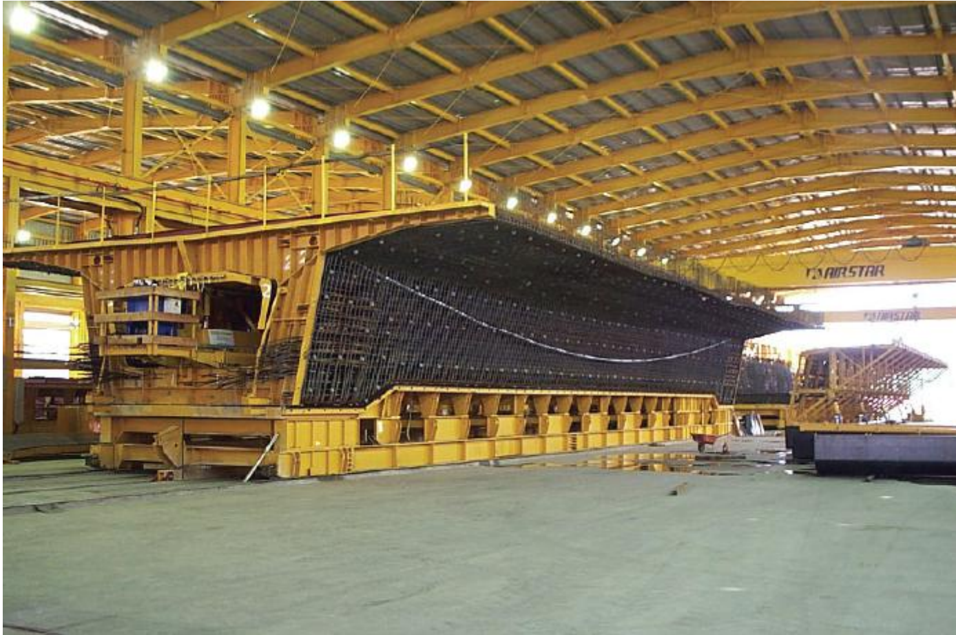
THE REBAR CAGE
