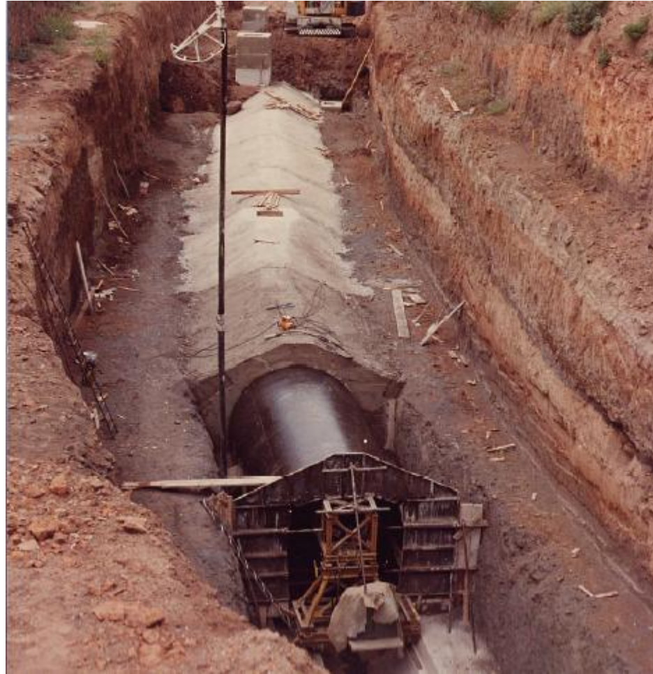
SMALL TUNNEL FORMS
