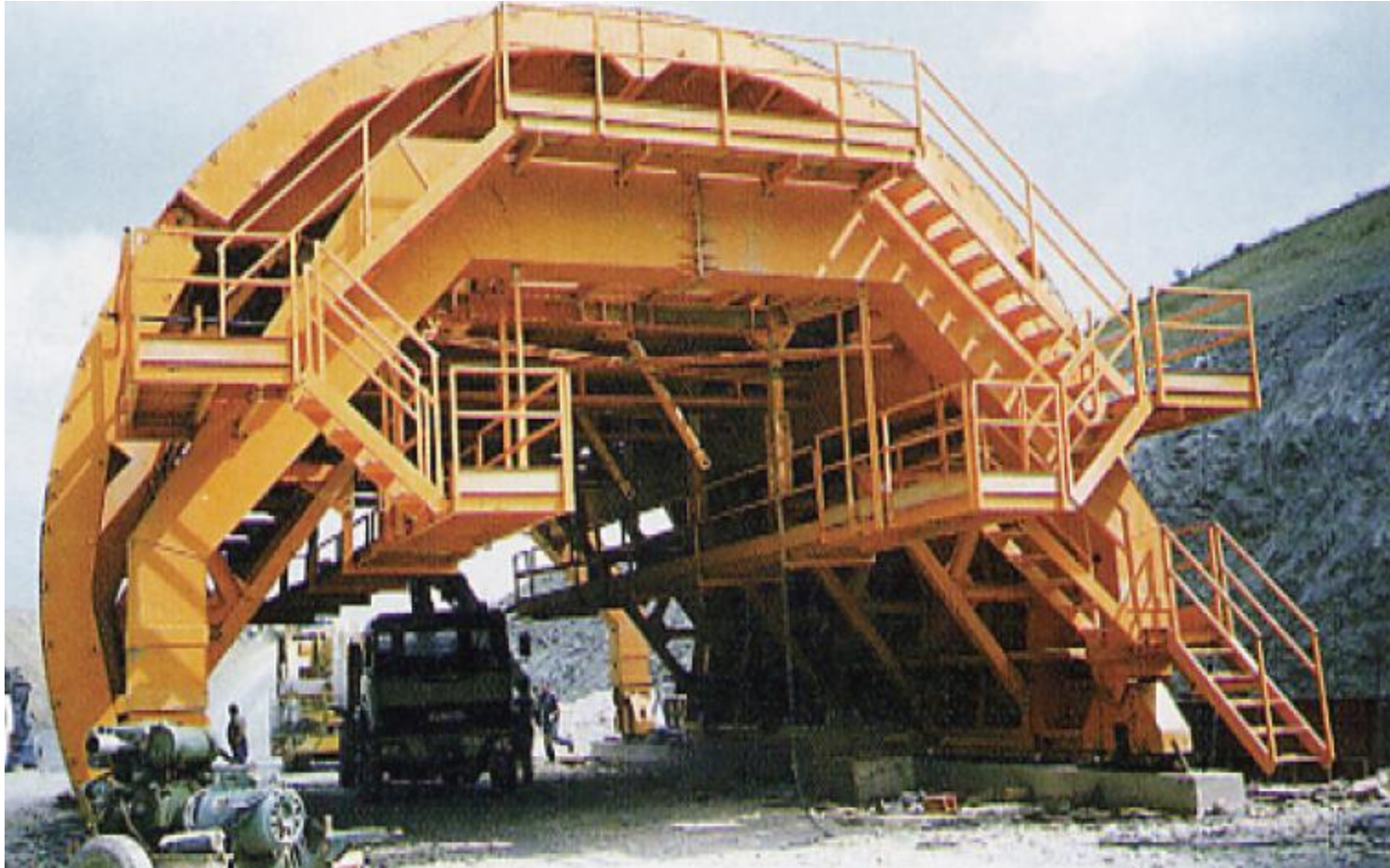
SELF- REACTING FORMWORK
