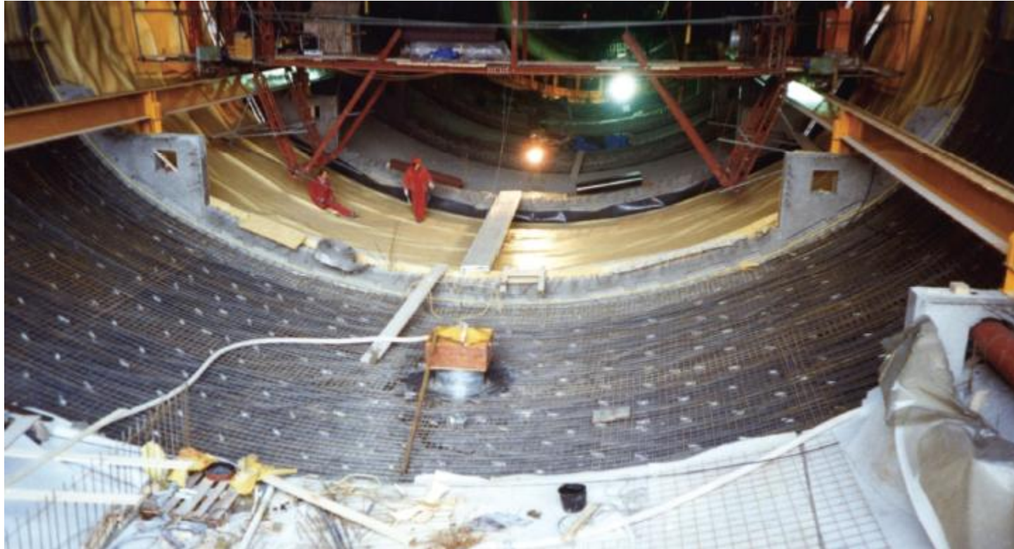
THE REBAR CAGE PREPARATION
