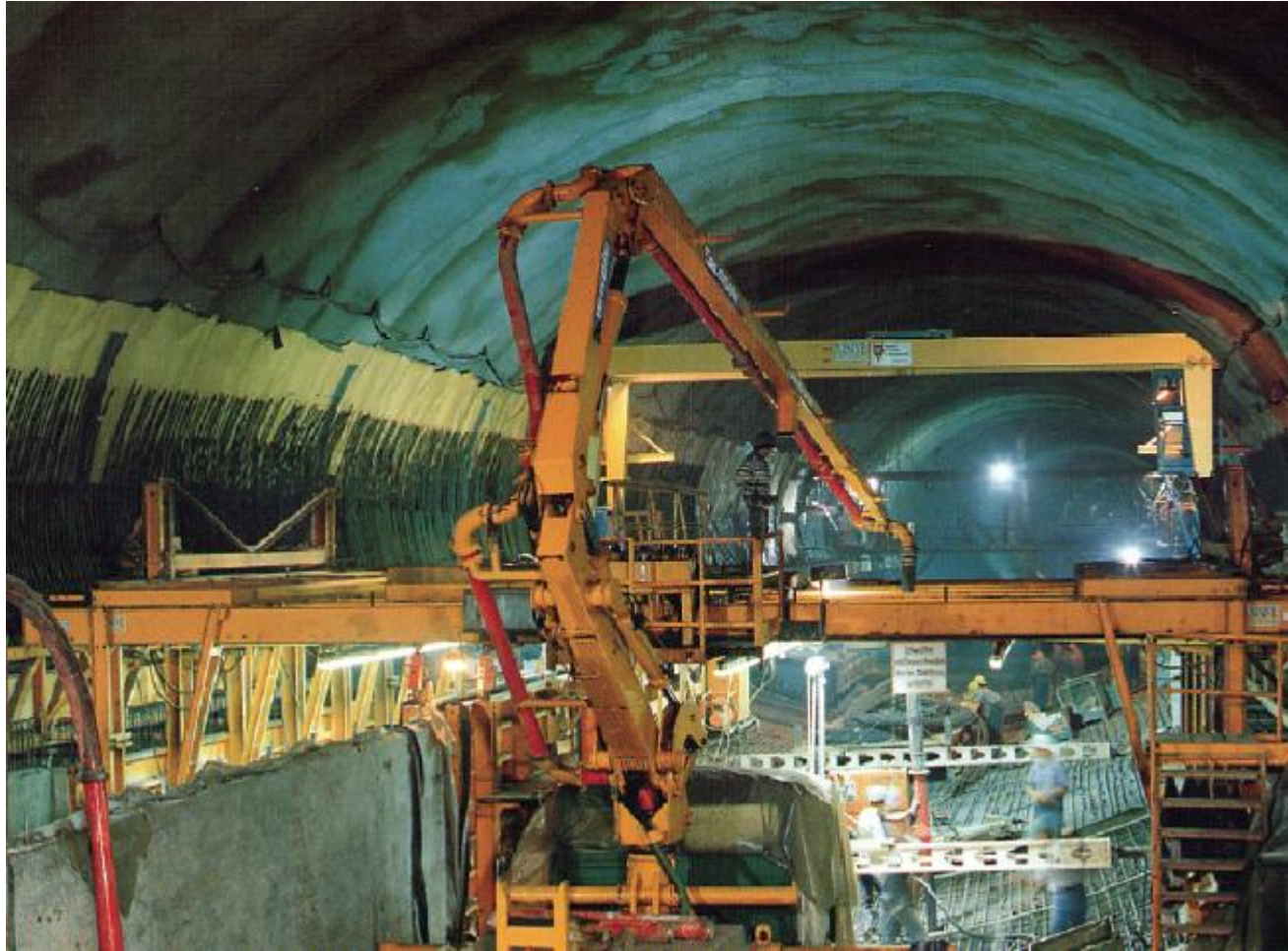
THE CASTING OPERATIONS
