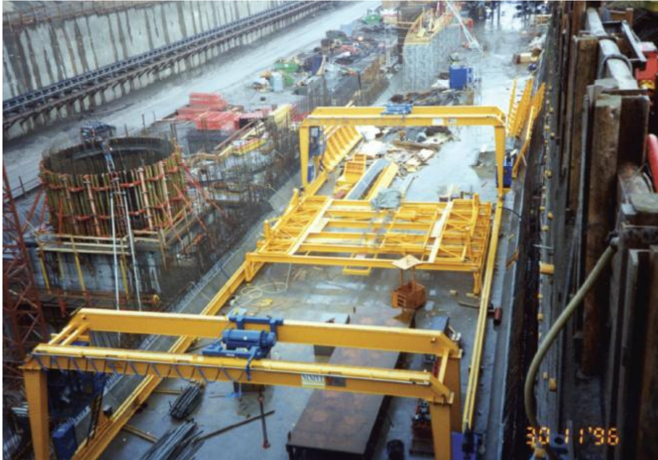
THE FORMWORK INSTALLATION
