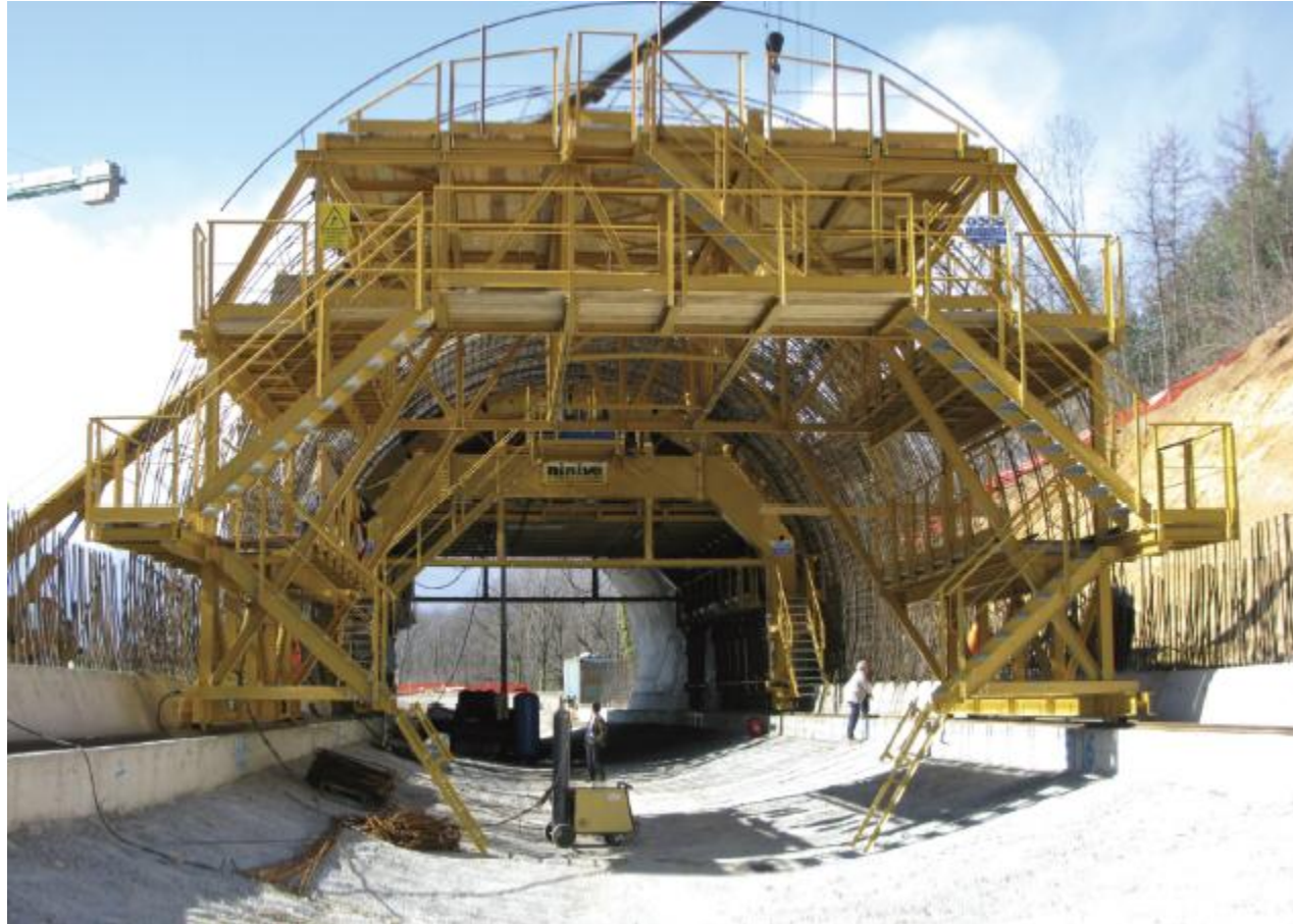
REBAR CAGE TROLLEY
