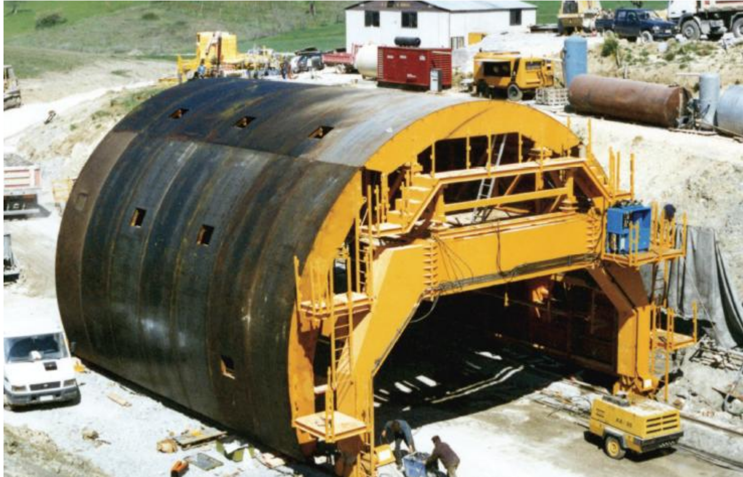
SELF- REACTING FORMWORK
