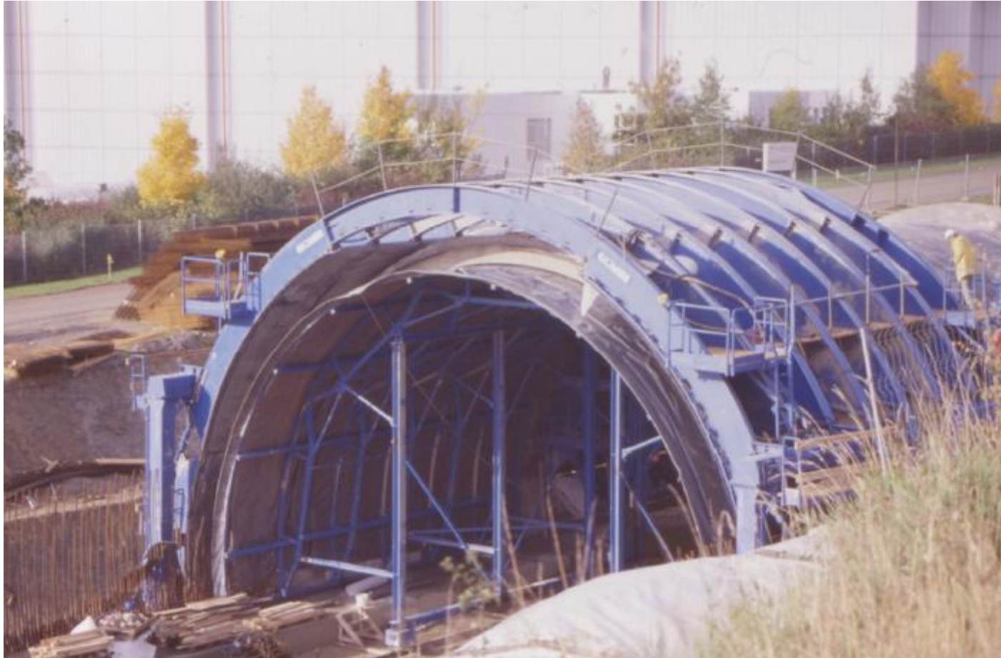
OUTER FORMWORKS
