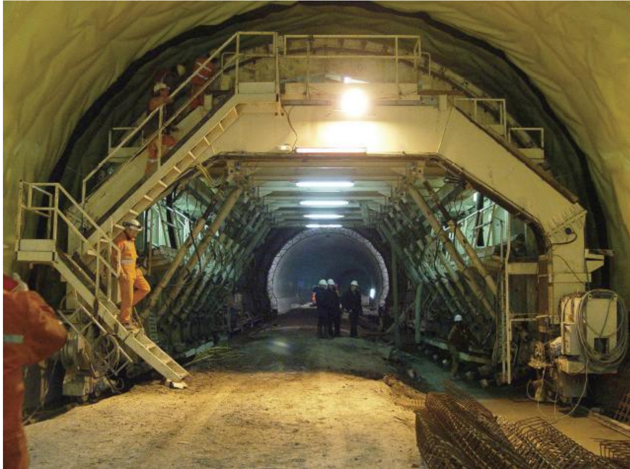
SELF- REACTING FORMWORK
