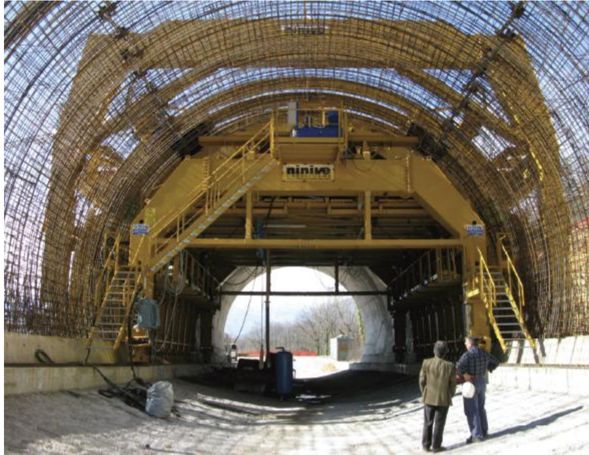
INTERNAL & EXTERNAL FORMWORK
