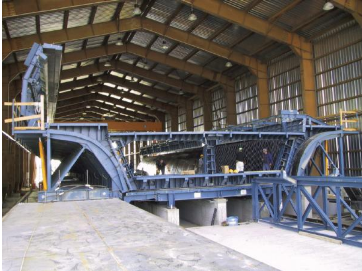
THE PRECAST AREA
