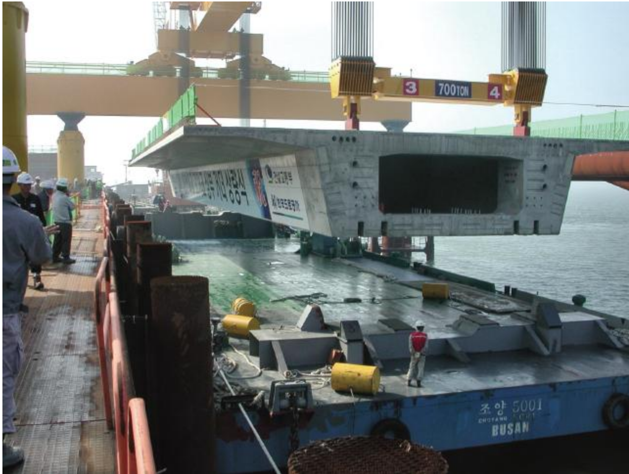
CONCRETE BOX GIRDERS
