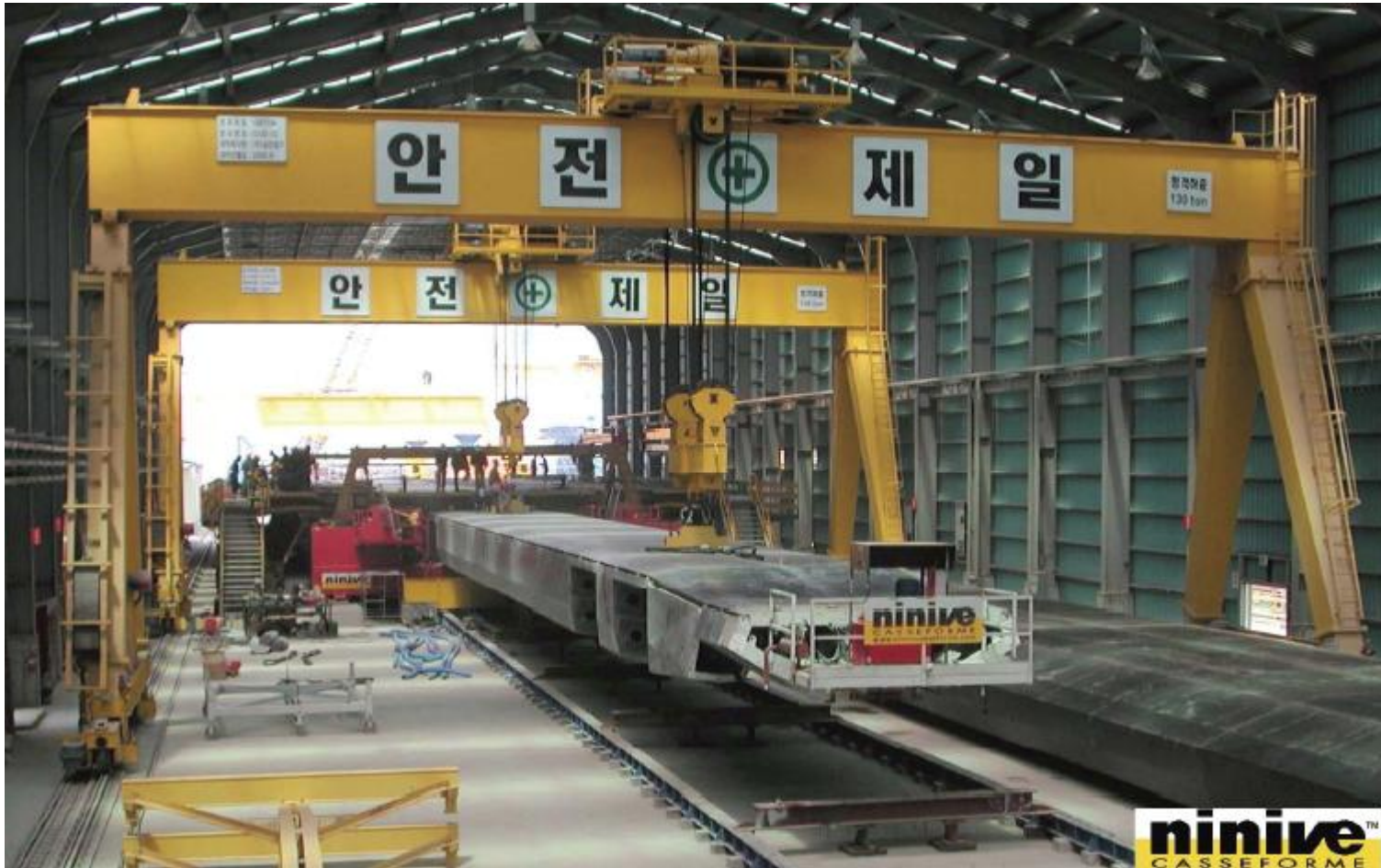
CONCRETE BOX GIRDERS
