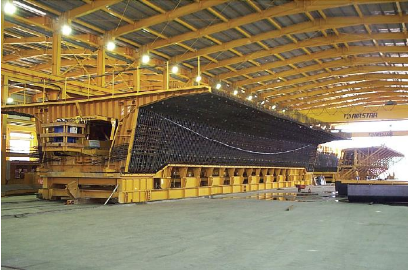
THE REBAR CAGE
