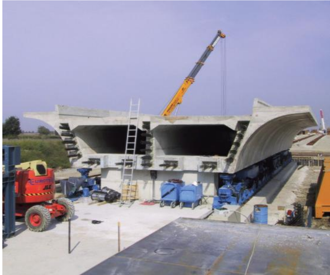
TWIN CELL BOX GIRDER
