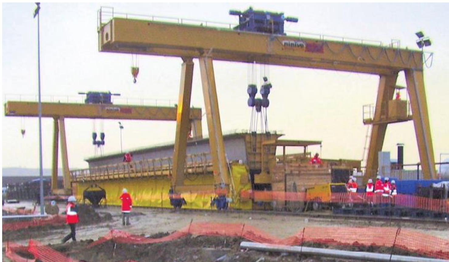
“U” SHAPE BEAM SELF REACTING MOULD
