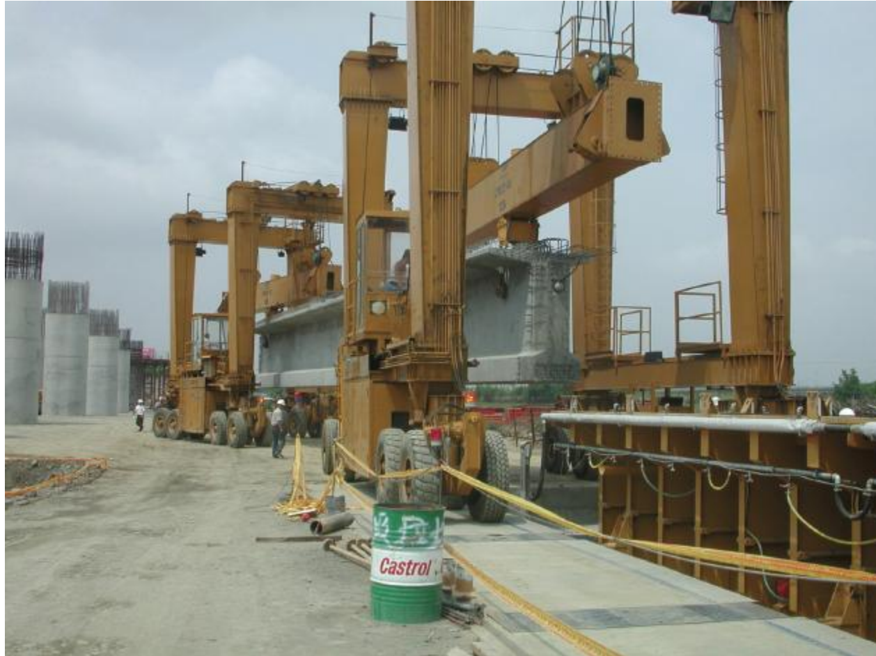
“T” SHAPE BEAM CONVENTIONAL MOULD & DRAWING BACK FLANKS
