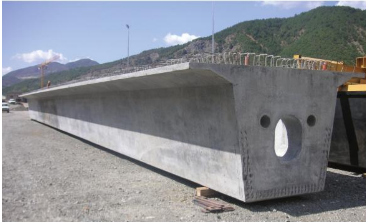
U SHAPE BEAM SELF REACTING MOULD
