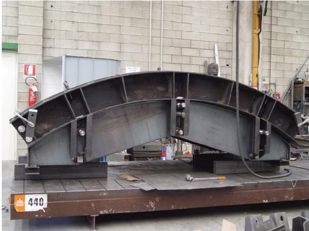
THE FORMWORK CONSTRUCTION
