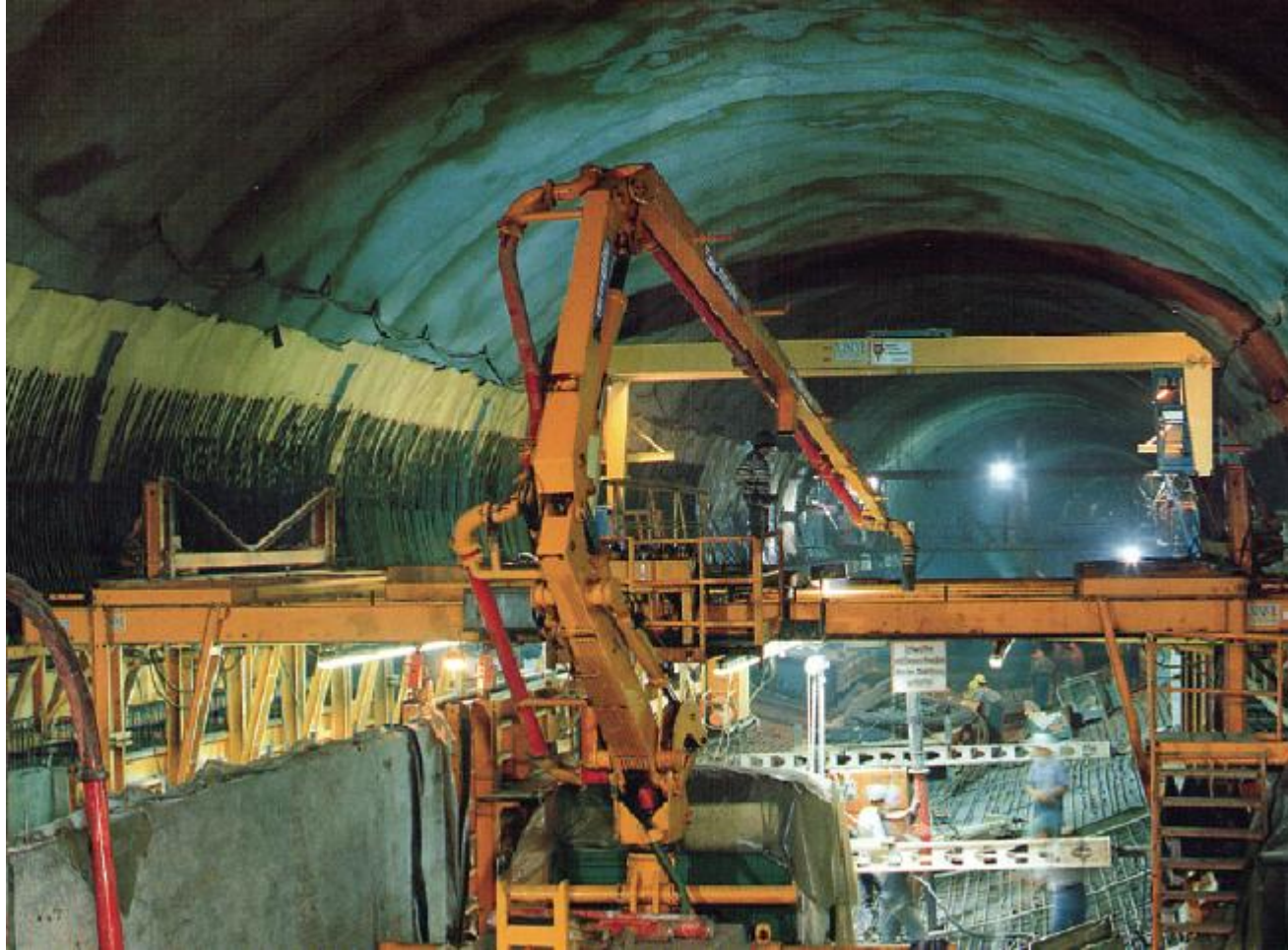
THE CASTING OPERATIONS
