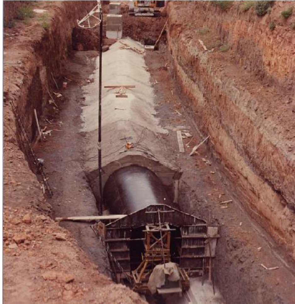
SMALL TUNNEL FORMS
