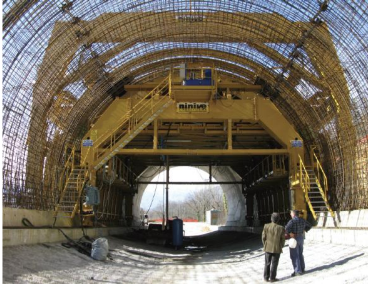
INTERNAL & EXTERNAL FORMWORK
