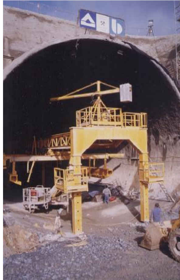
THE SELF LAUNCHING FORMWORK
