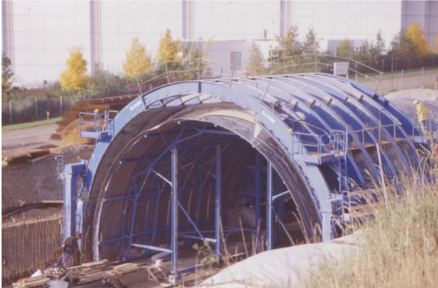
OUTER FORMWORKS
