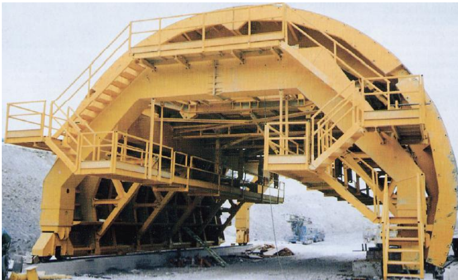
SELF- REACTING FORMWORK
